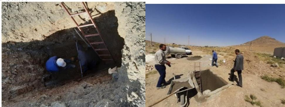
Figure 4: Excavation and control of the dam model within the ground and the completion of the earthen dam plaster.
